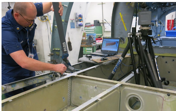
AMT1 Hansen using the FARO Quantum Arm to 3D to scan a recently replaced Nine Degree Frame on CGNR 6522.
