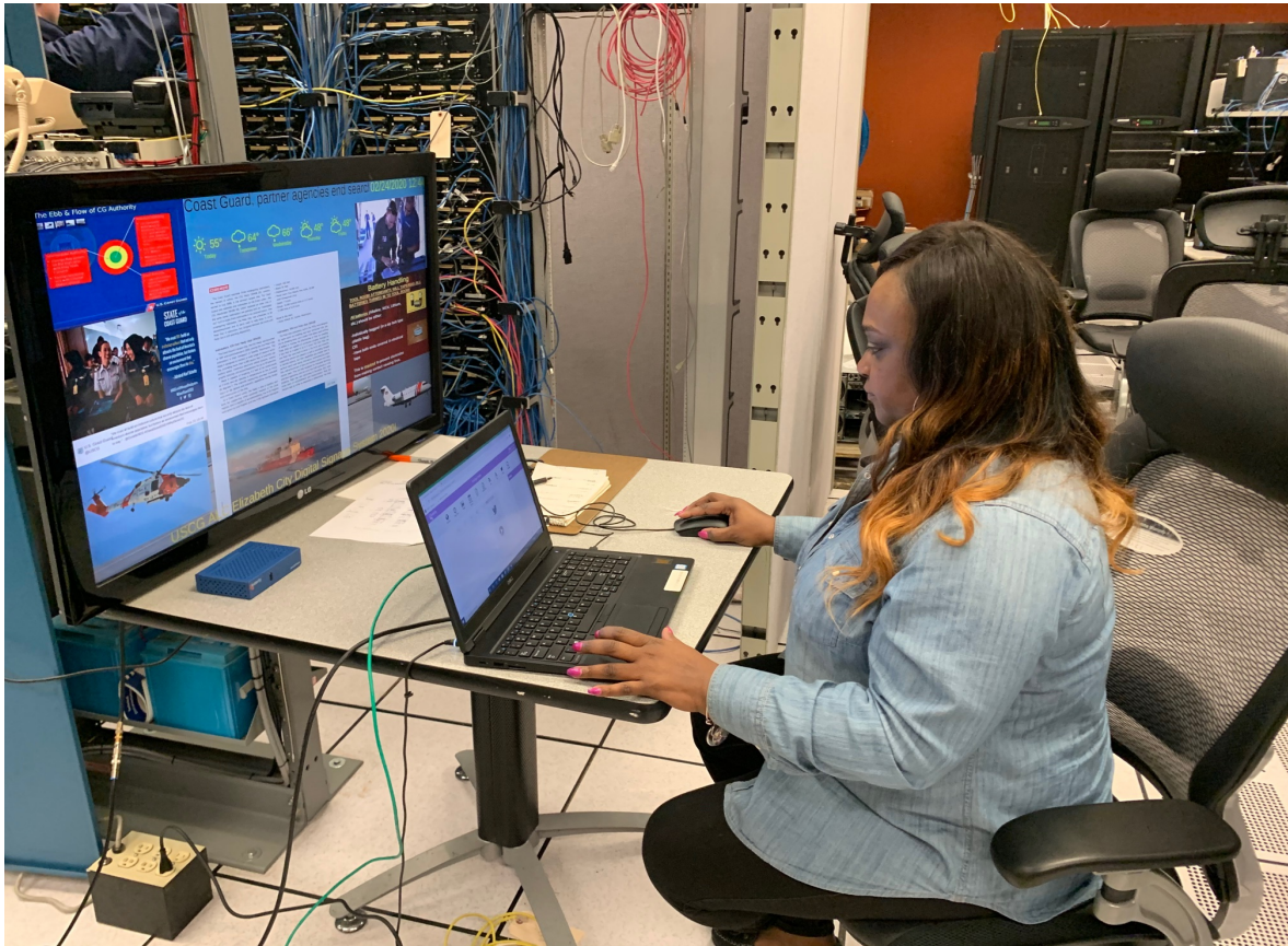
“Ms. Camie Proctor works on the ISD CCTV system within ISD’s Server Room”.
